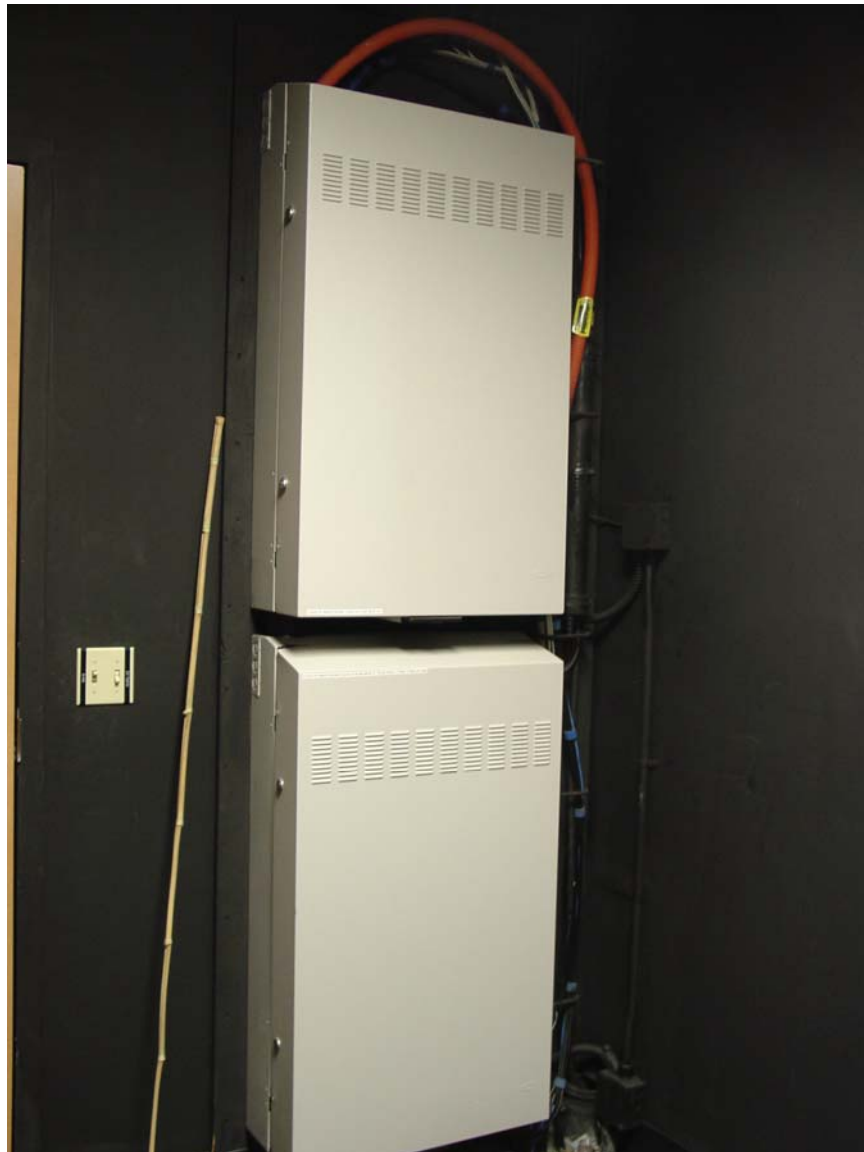
Figure 37 Type 3B Wall-Mounted Cabinet
